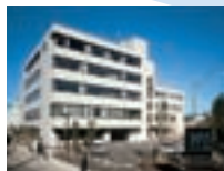
● Yokohama Engineering Center
