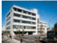
● Yokohama Engineering Center
