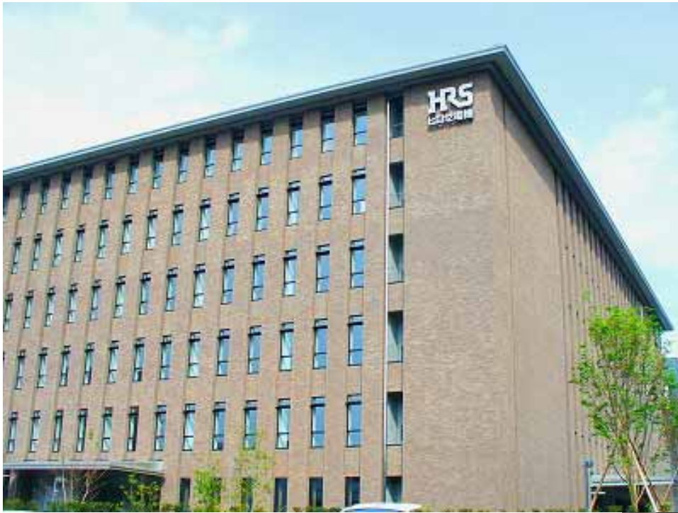
The Exterior of the Building
